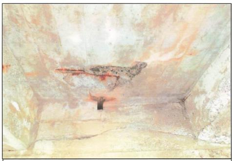
Photo 7: Spalling with Corrosion Staining in Soffit
