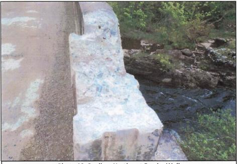
Photo 10: Spall on Northeast Barrier Wall
