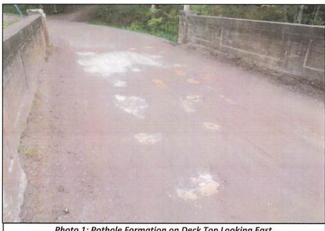
Photo 1: Pothole Formation on Deck Top Looking East
